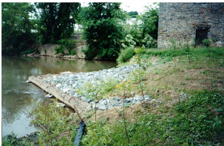
Photograph of a newly installed log frame deflector.
