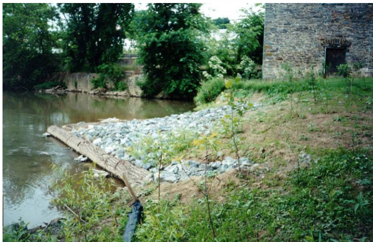
Sample photograph of a newly installed log frame deflector
