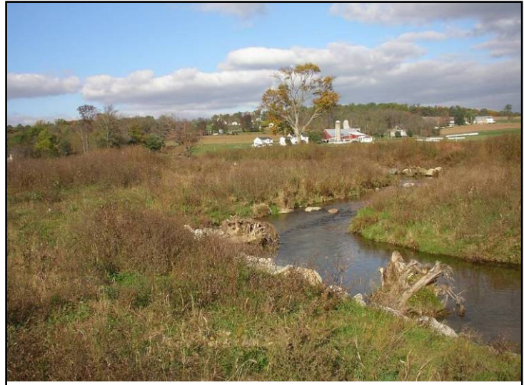
Established streambank stabilization project with root wads.
