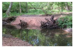
Root wads from clearing operations may be anchored into the streambanks to slow the flow of water in the stream and create habitat for fish and aquatic life. Log sections may be used to create vanes and deflectors to protect banks and create in-stream habitat. Where needed, boulders can be placed either randomly for fish habitat and to disperse
