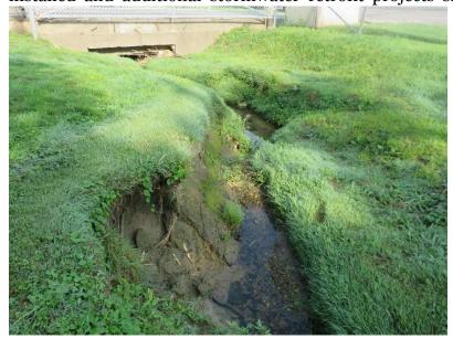
stream channel, grading to create floodplain capacity and stable, vegetated streambanks should be completed. The riparian zone should then be planted with native vegetation. Within the stormwater swale that discharges to the stream from the south, a regenerative stormwater convevance installation that retains and filters stormwater through a compost/ sand bed between constructed riffle areas should be installed.
