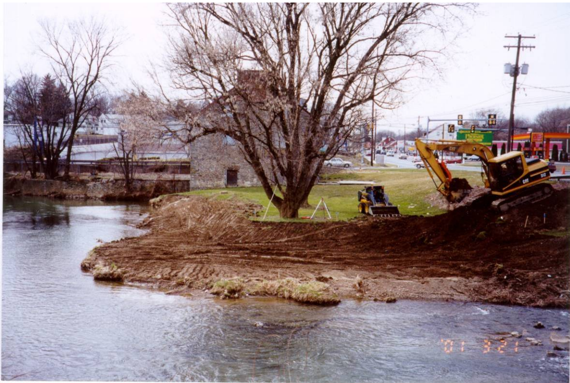
Sample photograph of floodplain restoration – removing previously placed fill and legacy sediments
