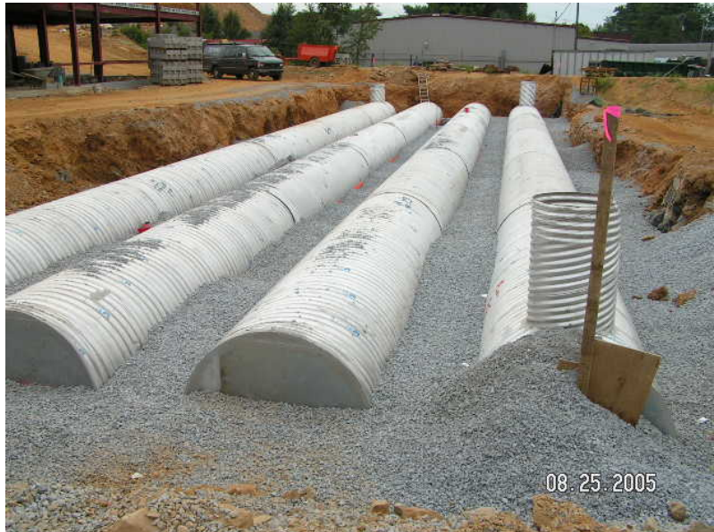
Sample photograph of an underground detention facility installation
