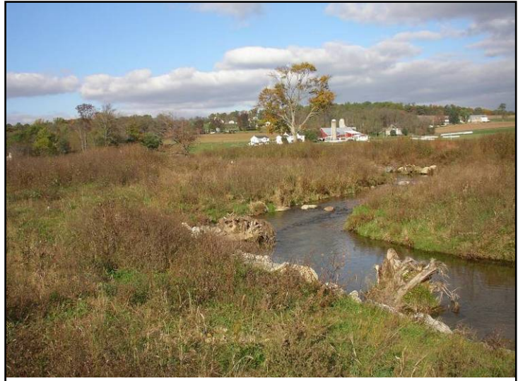
Established streambank stabilization project with root wads.
