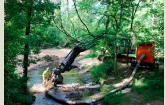
Excavation and pumping at Nixon Park
