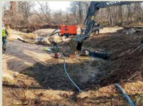
Stream bank grading on Plum Run Phase 1, December 2019
