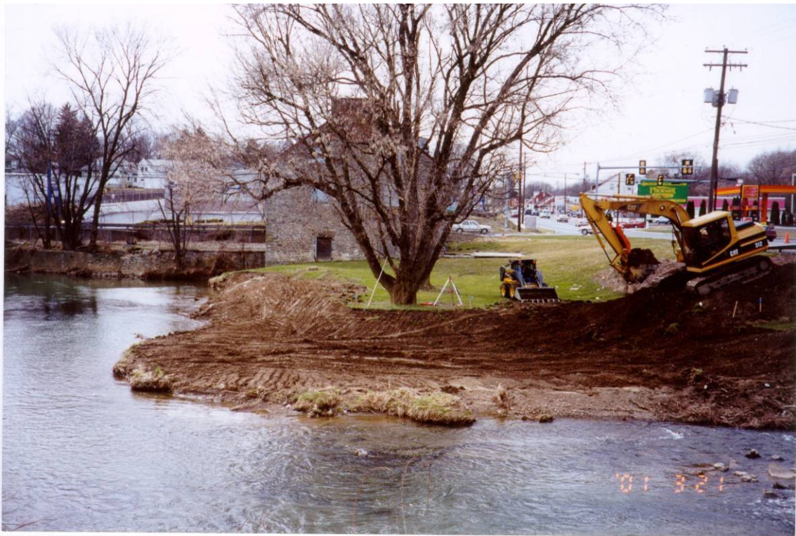
Photograph of floodplain restoration – removing previously placed fill and legacy sediments.
