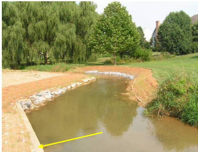
Photograph of a mudsill indicated by the yellow arrow.
