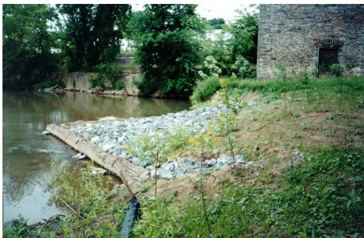
Photograph of a newly installed log frame deflector.
