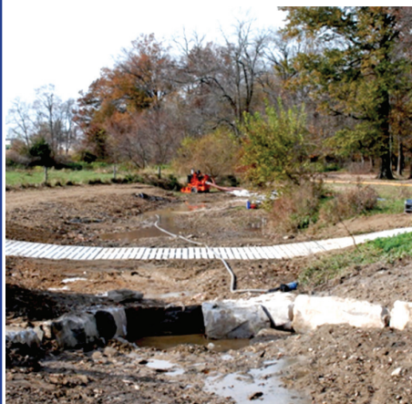
Cross vane and livestock crossing installation
