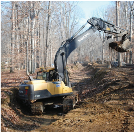
Streambank grading
