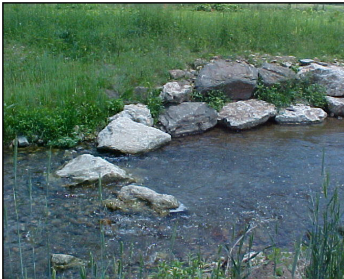
In-stream structures such as this J-hook can be installed to minimize erosion of the newly restored streambank until vegetation becomes established.
