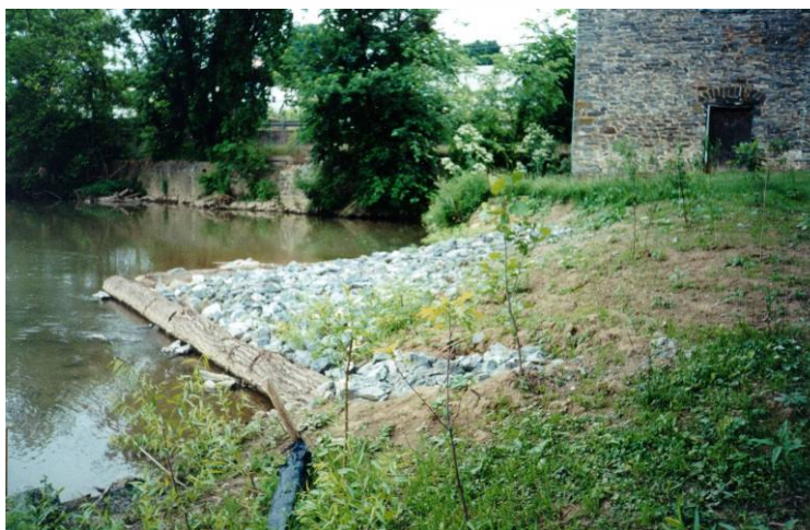
Sample photograph of a newly installed log frame deflector
