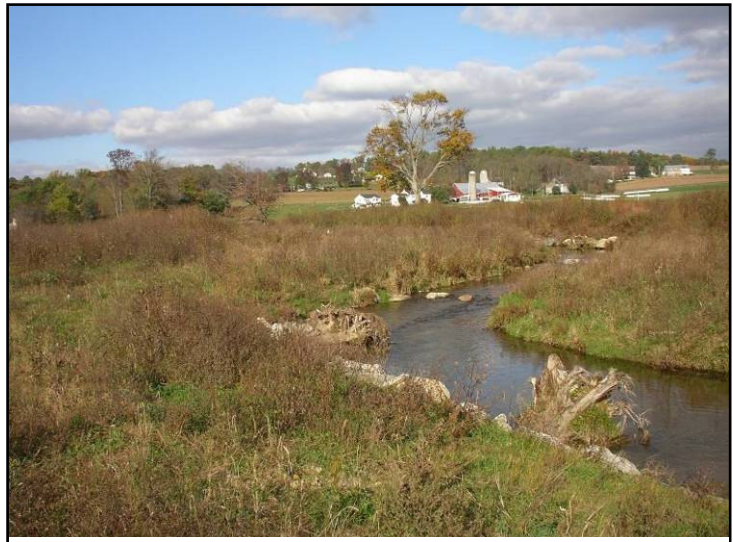
Established streambank stabilization project with root wads.
