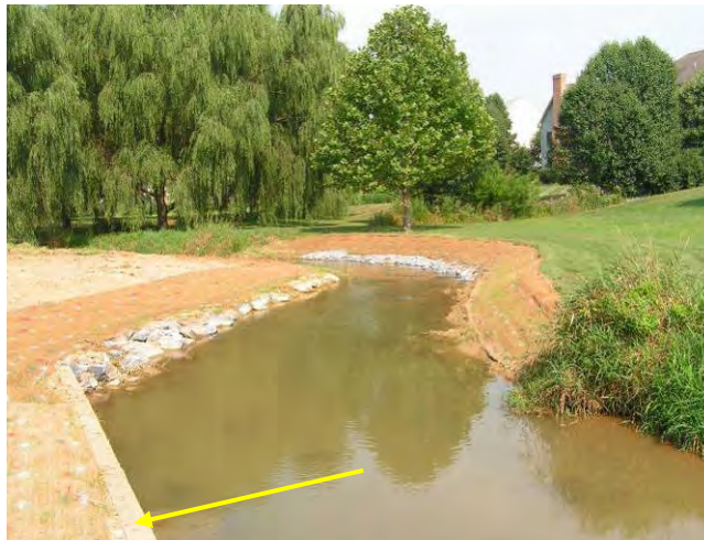
Sample photograph of a mudsill indicated by the yellow arrow
