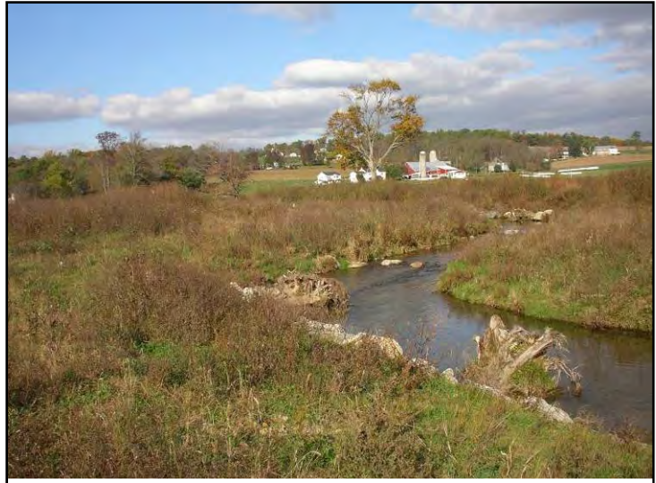
Established streambank stabilization project with root wads.
